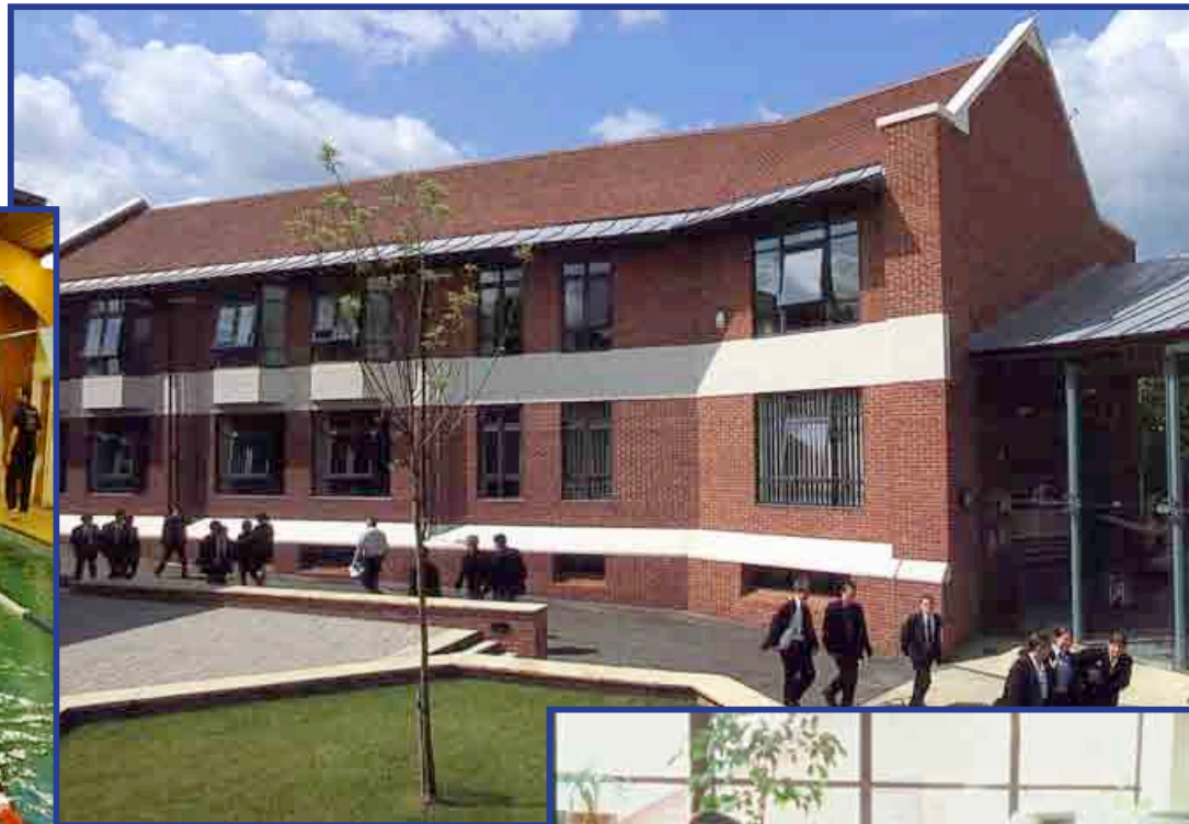
Mackinder Building classrooms
