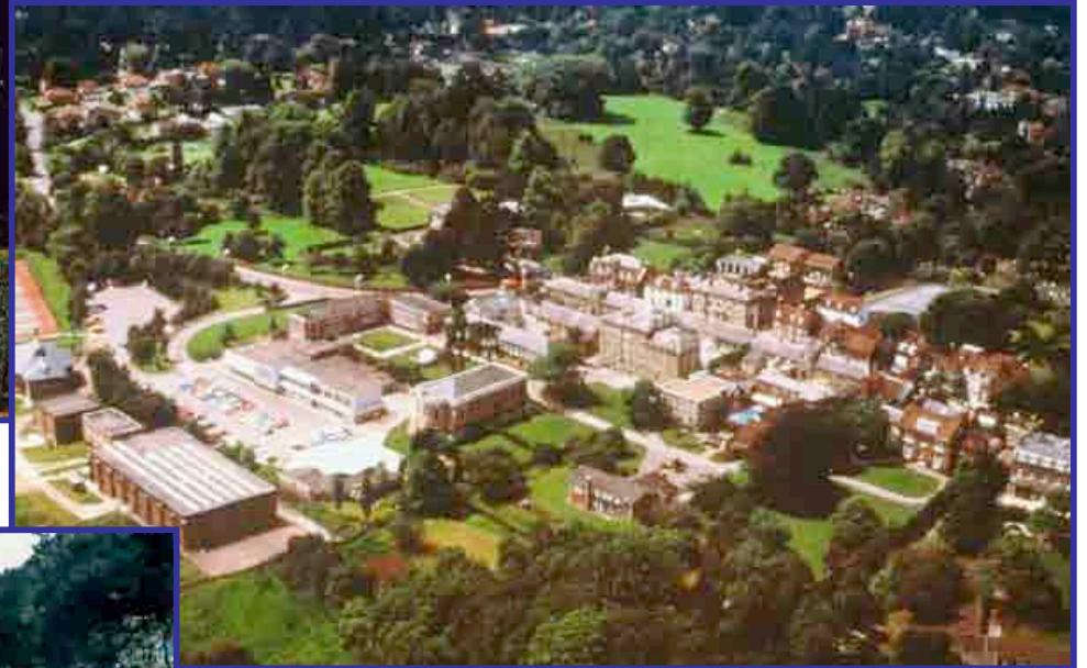
Aerial view of school
