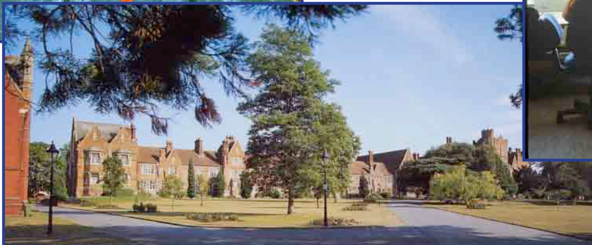
View of the main school buildings
